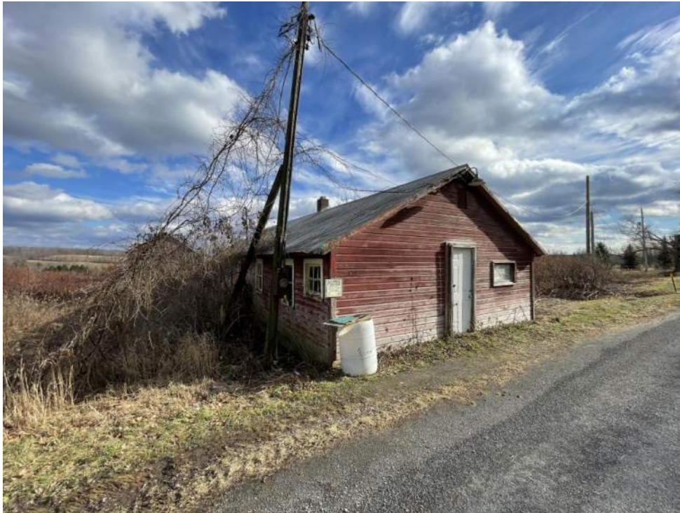
View of on-site structure at intersection of Tucker Road and Aiken Road.
