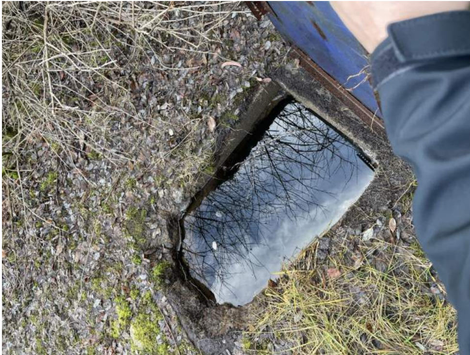
View of pit positioned beneath concrete at entrance filled with stormwater.
