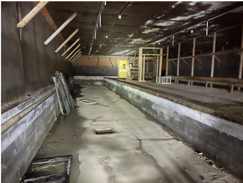
Typical view inside barn.
