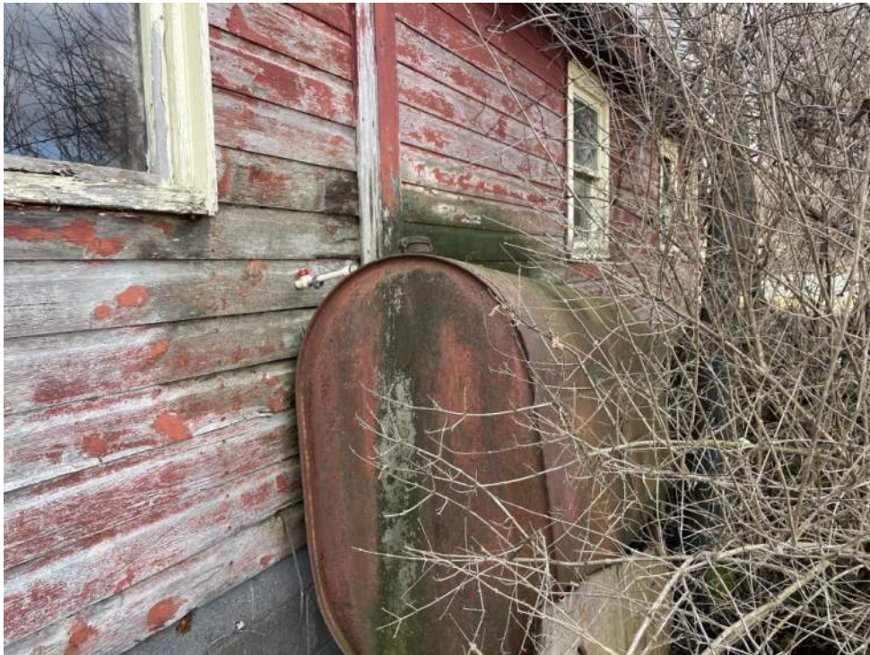
Empty 275-gallon fuel oil AST associated with above noted structure. Evidence of release was not observed.
