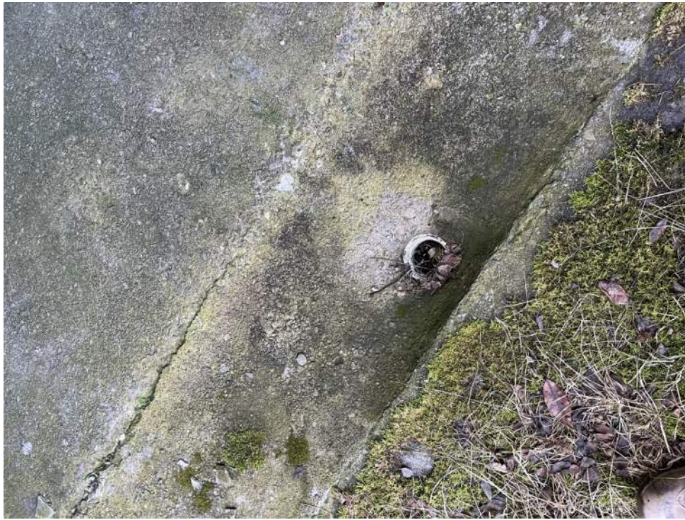
Typical view of drain leading to entrance pits.
